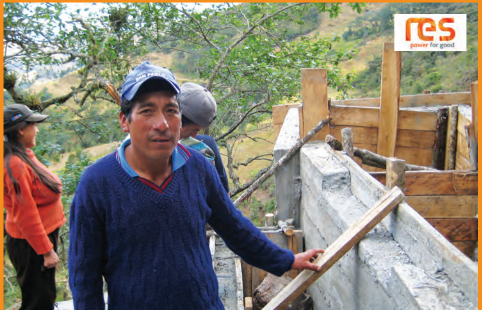
CESAR HUAMAN BUILDING THE MICRO HYDRO PLANT IN PERU
