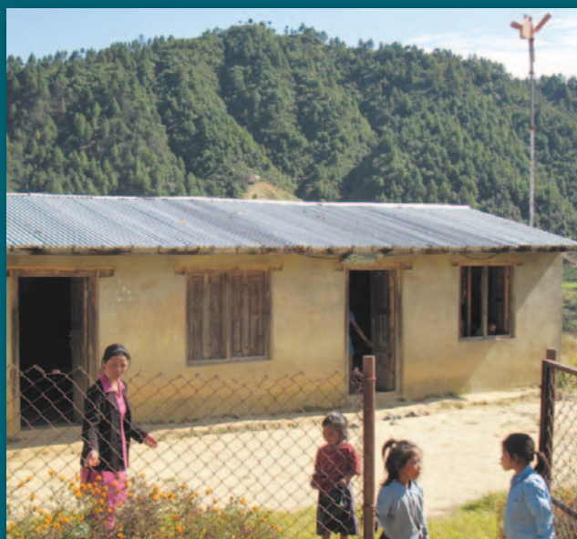
SCHOOL IN NEPAL POWERED BY WIND TURBINES ▶
