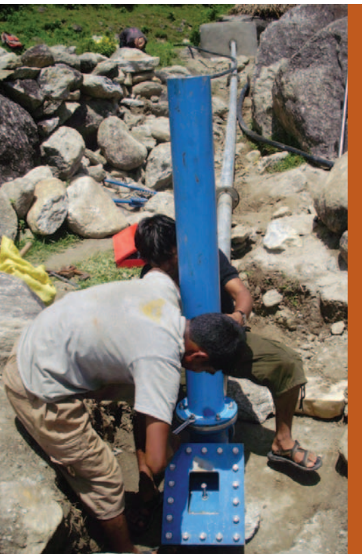
Ram pump installation
