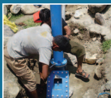
4-5 PUMPING WATER IN NEPAL
